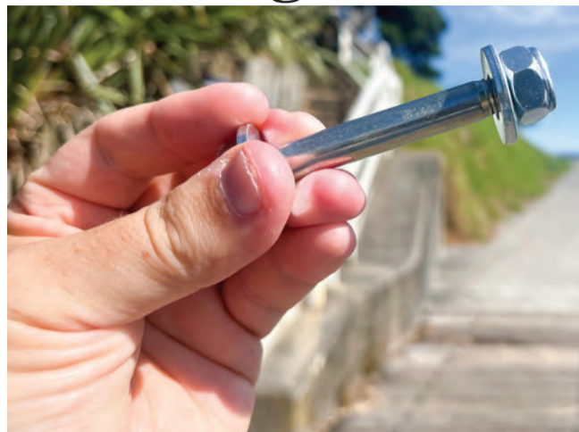
Bolt thefts are putting the public at risk.
