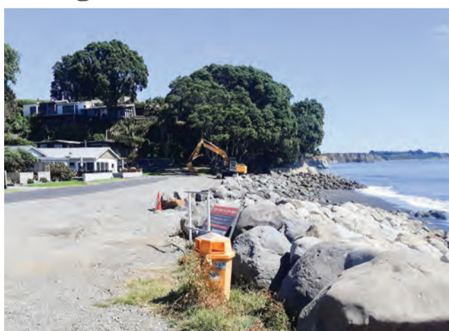
400 tonnes of rock have boosted the Onaero Beach seawall
