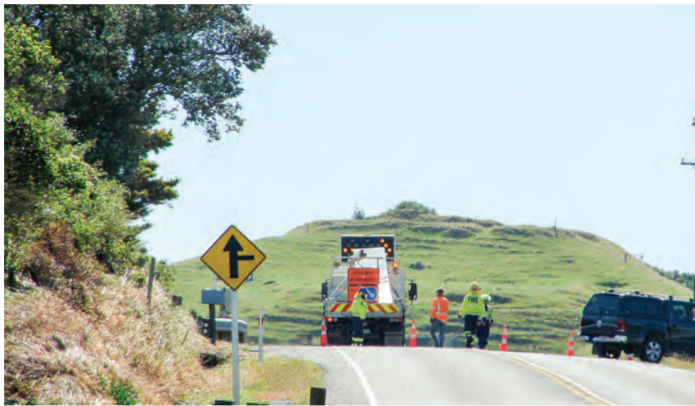
Roadblock just north of the bridge over the Warea River (Taikaparua) on State Highway 45.
